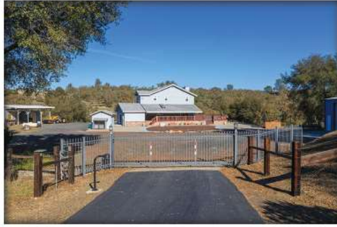
ELECTRIC SECURITY GATE
